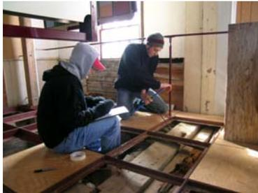
the wood. The operator then took an extractor and removed the core from the borer and placed it into a clear plastic tube that was immediately labeled. A description of the area, type of wood, and setting was depicted on a log sheet. The
