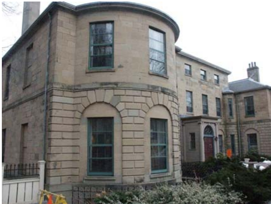
Figure 1: The Government House in Halifax under renovations, January 2008. Photo: B.E. Phillips
